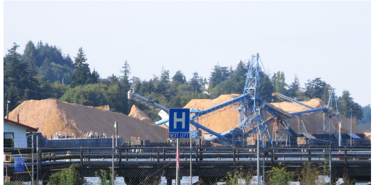
Typical Chip Pile in Coos Bay, Oregon
